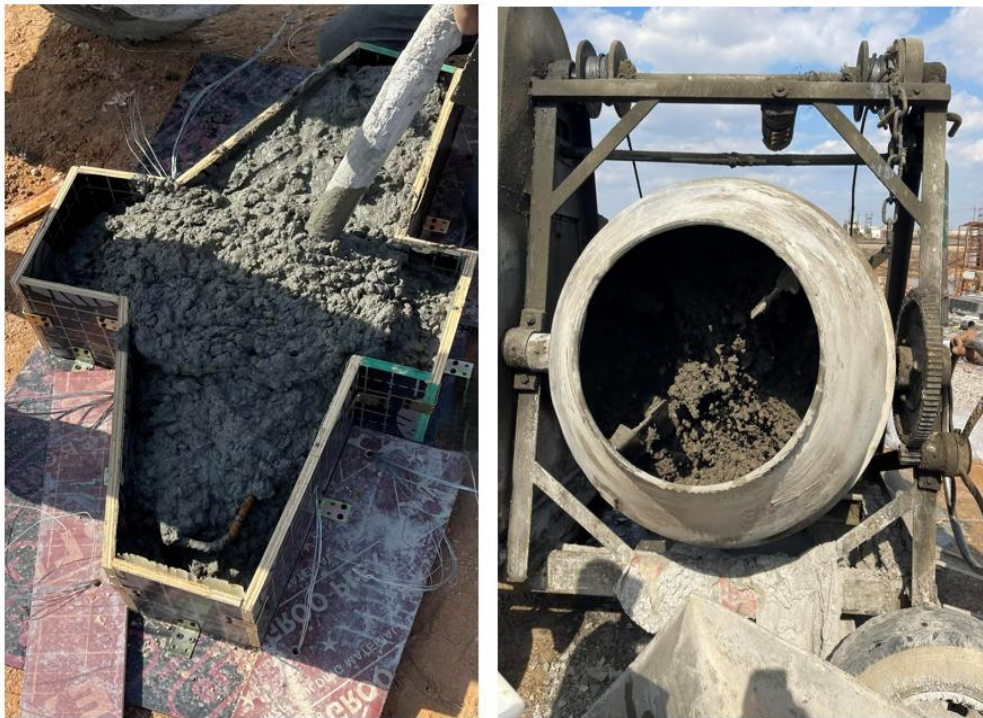
Figure 3. Mixing process showing the use of the vibrator
