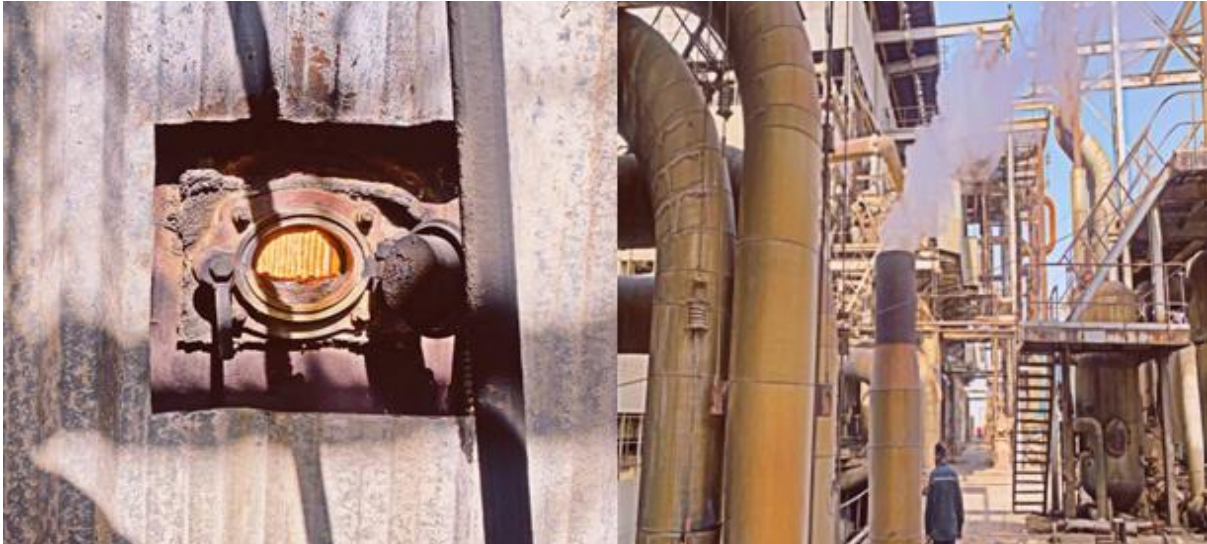
Figure 4. Bottom ash production in a thermal power plant
