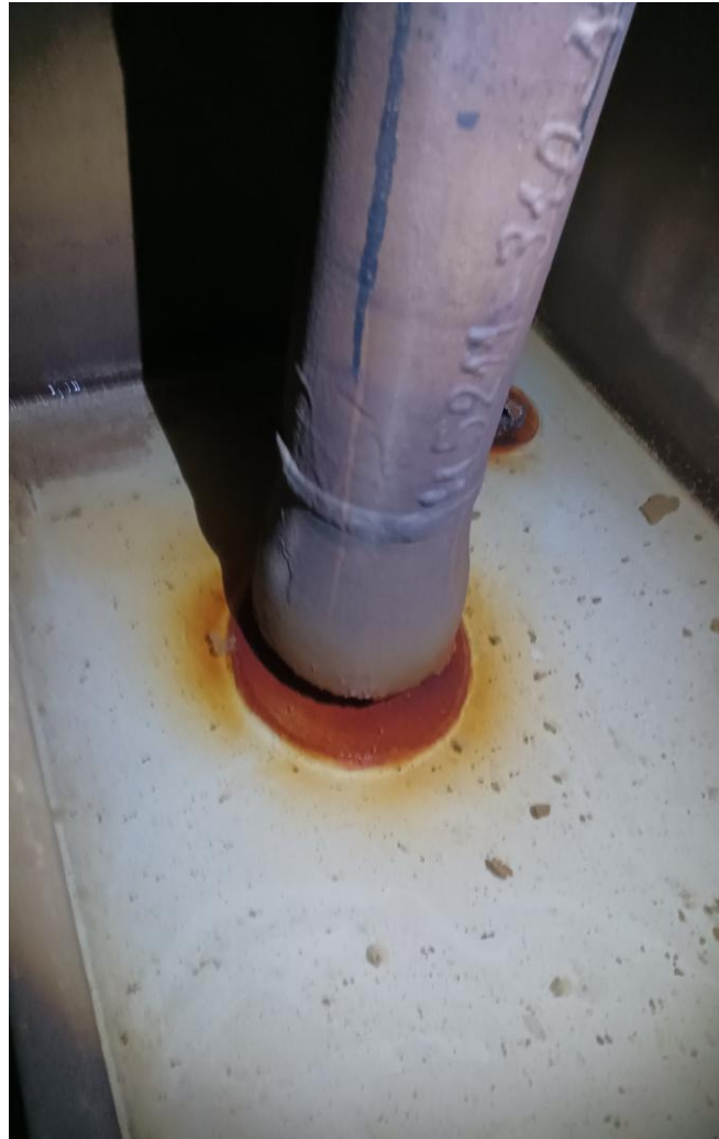
Figure 2. Option two with installed plate
