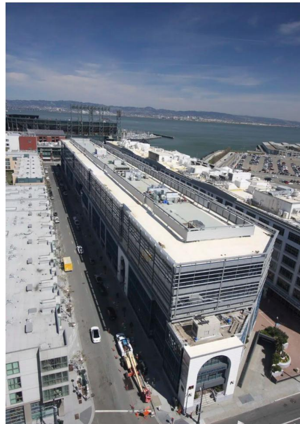
After the superelevation
