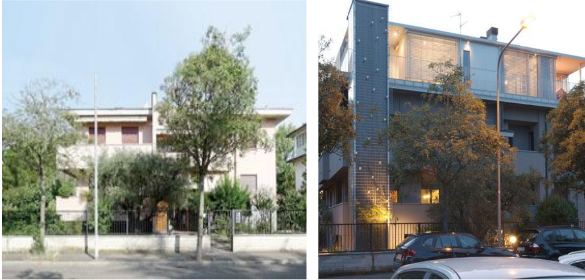
Before the superelevation
